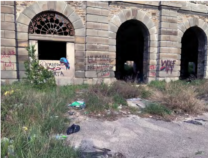
Fig. 2: The occupied Silos in 2024
